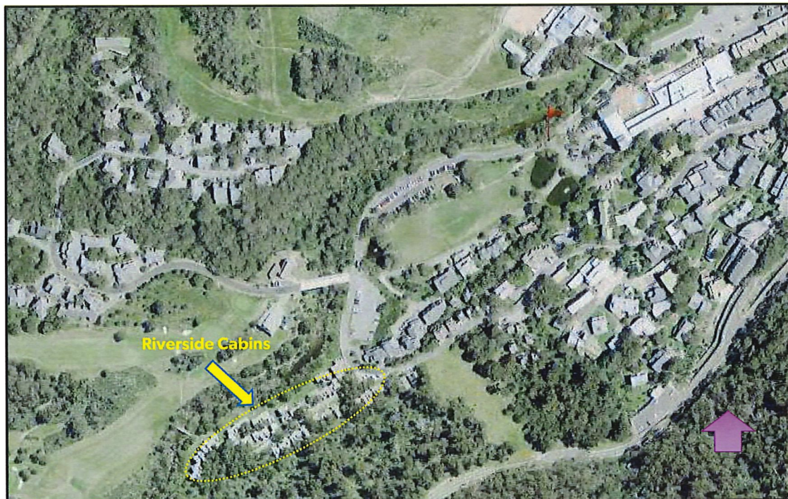
Figure 1: Riverside Cabins location in context to Thredbo Village (Source: SIX Maps 2018)
